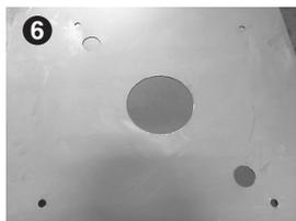
Open the holes around the marks, with a hole saw, etc.
