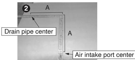
Mark the center of one of the drain pipes, at the distance from the mark made in 1 specified in the installation dimensions on pg. 2.
