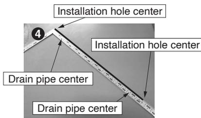
Mark the centers of the installation holes (x 2), along the line drawn through the marks made in 2 and 3.
