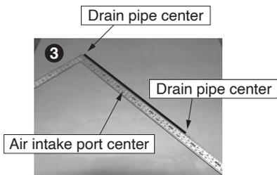
Mark the center of the other drain pipe, along the line drawn through the marks made in 1 and 2.
